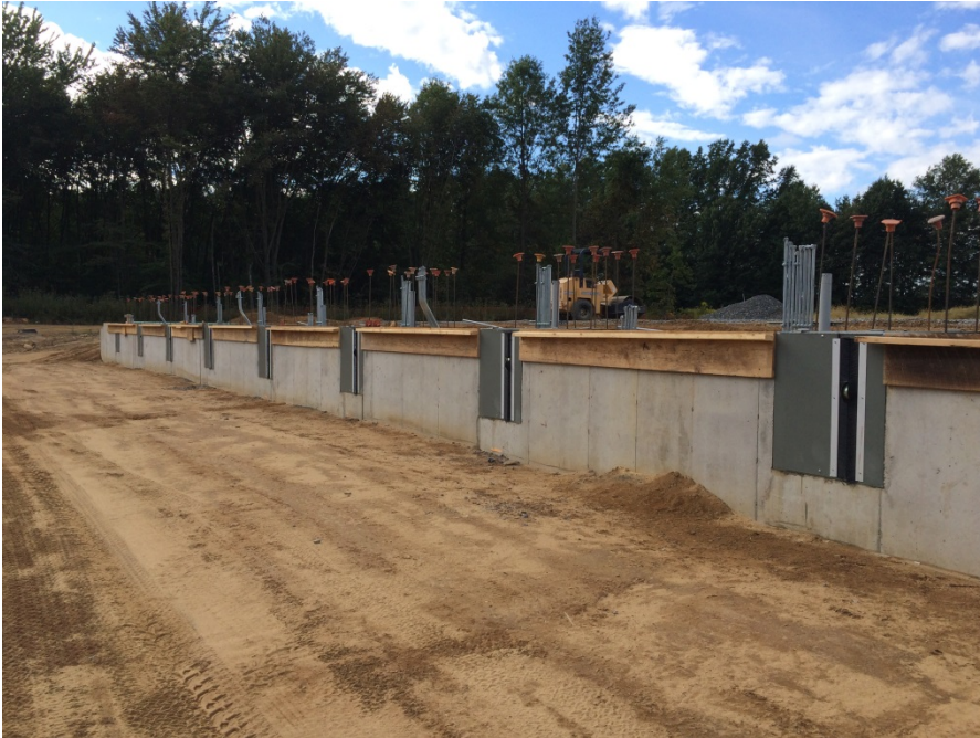
Prepare front wall with lumber form for Floor Pour & Front Angle Iron
