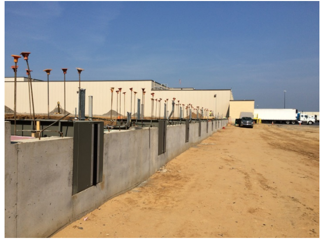
Prepare front wall with lumber form for Floor Pour & Front Angle Iron
