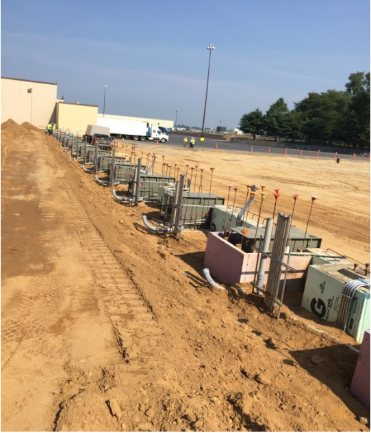
Conduit & Chases installed per drawings:
