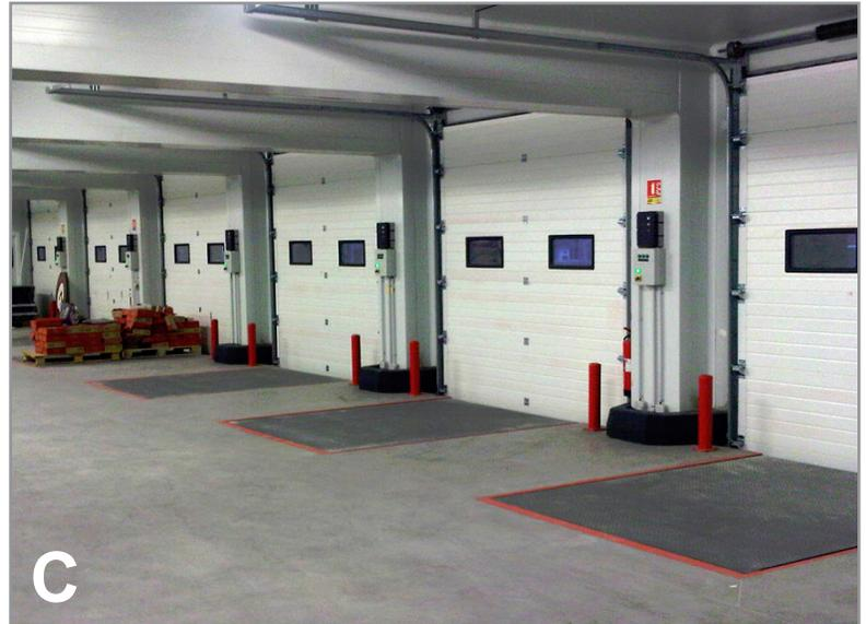
To comply with the new walking-working surface regulations, an employer is required to either equip their dock equipment with run-off guards or demonstrate that no risk for transfer vehicles to run-off the dockboard edge exists. LODEM recommends that employers utilize dockboards or dock levelers that comply with ANSI MH30.1 and ANSI MH30.2, respectively. Furthermore, when dock levelers without run-off guards are used,
